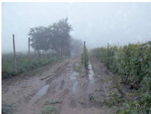
Figure 3. Consequences of heavy rainfall and the fog phenomenon in July, 2014
