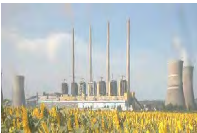
Fig. 1. The Turceni Steam Power Plant
