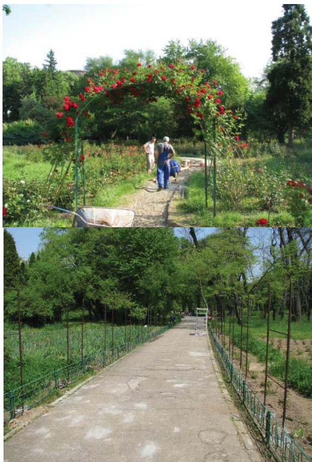
Fig.6. Aspects from the rehabilitation of the aisles and the construction of arches (orig.)
